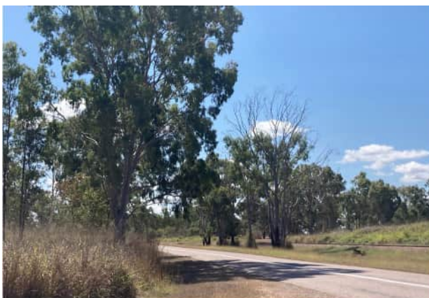
Plate 1 VP 1: Ayr-Dalberg Road Viewshed: View of the substation (looking north)
