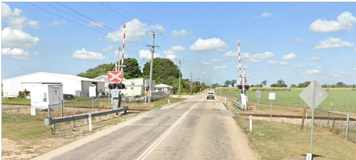
Figure 9 North Coast Line Rail Crossing of Ayr-Dalbeg Road
