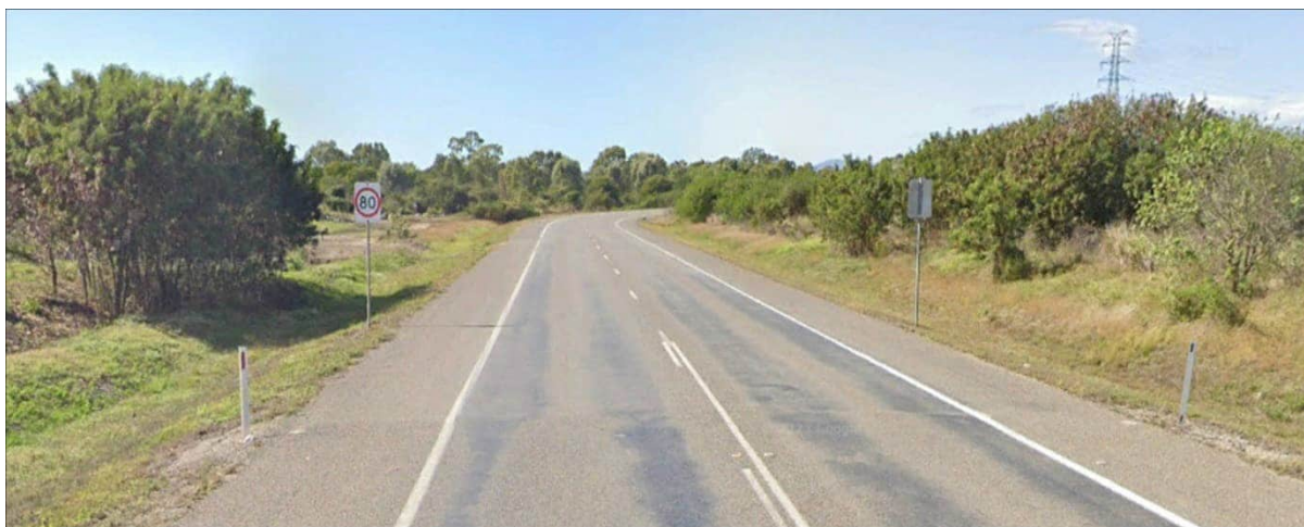
Figure 5 Townsville Port Road
