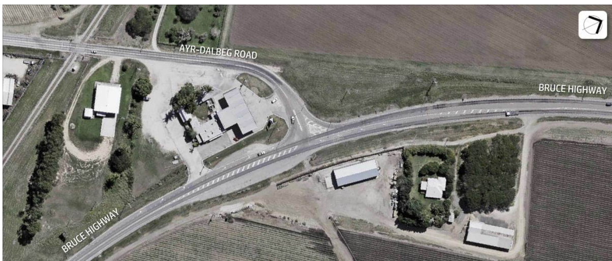
Figure 8 Bruce Highway / Ayr-Dalbeg Road Intersection – Existing Configuration
