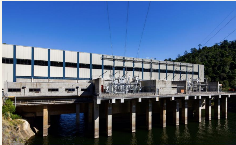
Hydro Plant – Pump, Sync Con Modes
