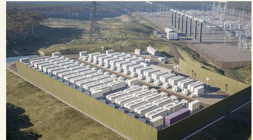
Grid Scale Batteries
