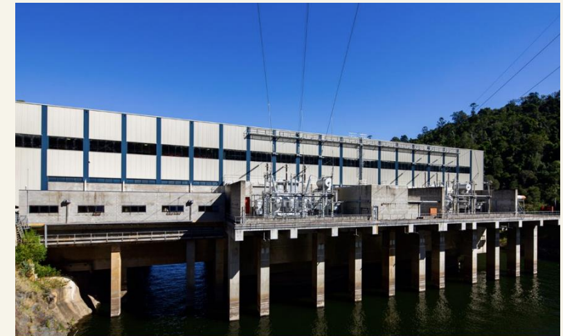
Hydro Plant – Generator
