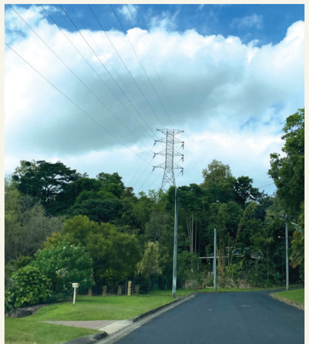
Existing transmission line between Redlynch and Woree
