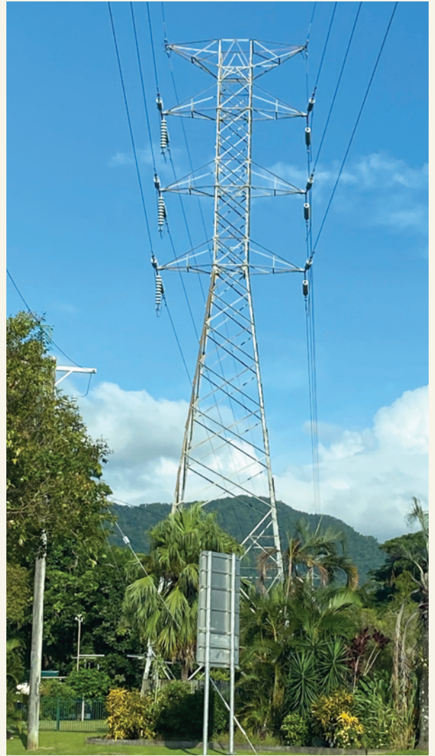
Existing transmission line between Redlynch and Woree
