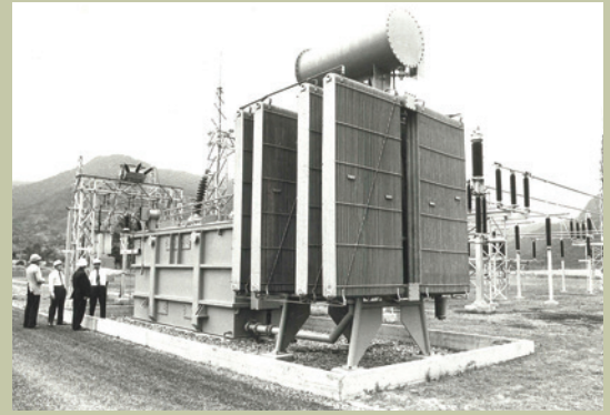
Kamerunga Substation - 1976 (Source: Powerlink archives)
