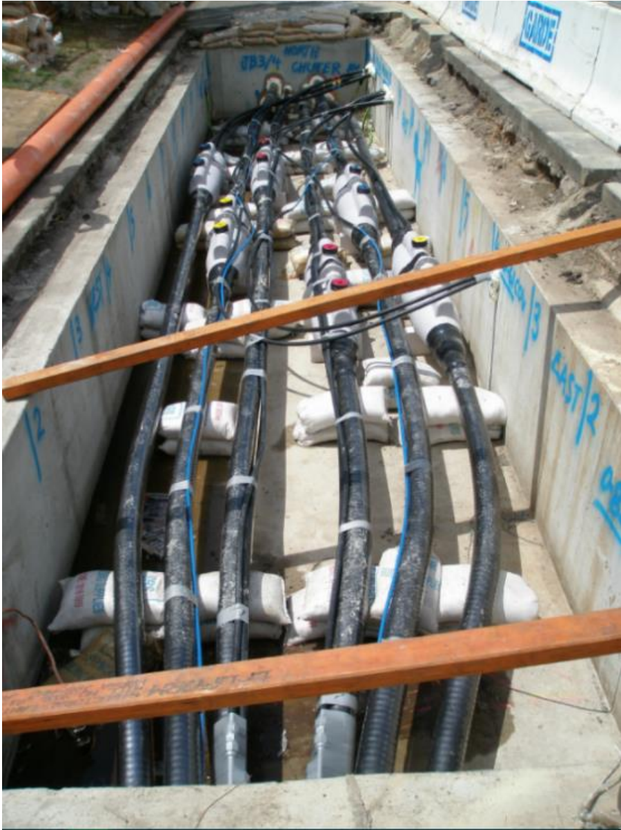
Figure 2-2 Example of a joint bay under construction
