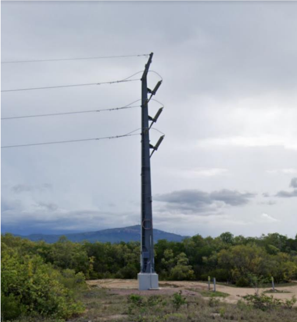
Figure 2-3 Example of an underground to overhead structure
