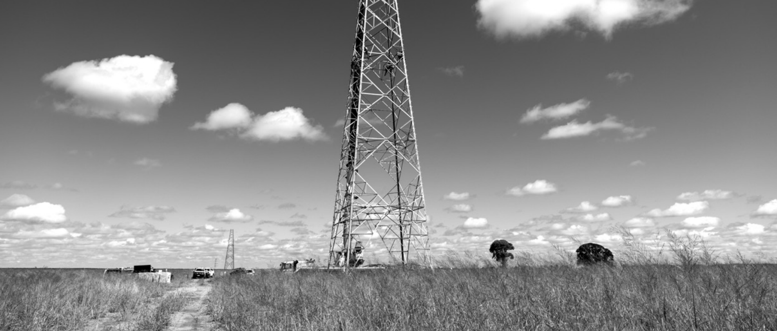
Work on the easement for the Wambo Wind Farm Connection Project, which is under development near Jandowae in the Western Downs.
